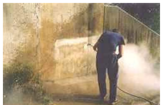
FINISHING REMOVAL OF GRAFFITI
