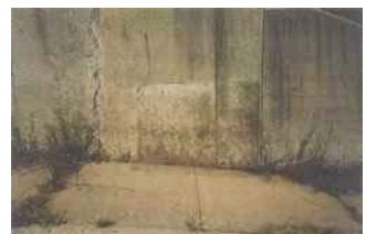
EIGHT HOURS AFTER COMPLETION NO EVIDENCE OF GRAFFITI
