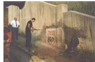
USING HOT WATER AT 3000 PSI TO REMOVE GRAFFITI
